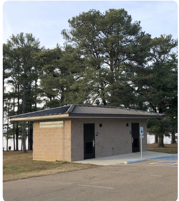
Restroom Facility at Ross Barnett Reservoir
